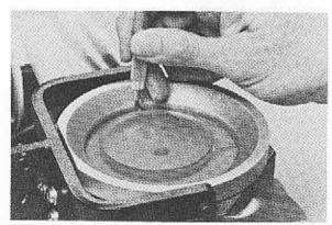
Then holding the cutter in a vertical position, trim tape by guiding the cutter around the outside edge of lens.
